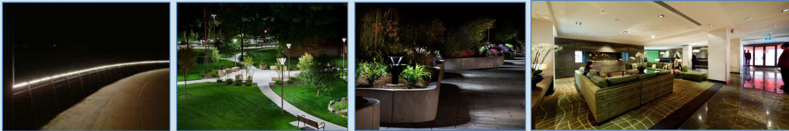
Figure 8: LED Lighting Schemes
